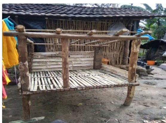
Poultry coup under construction
