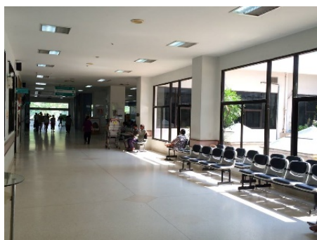
Figure 20. The current condition of the main corridor and the cashier counter
