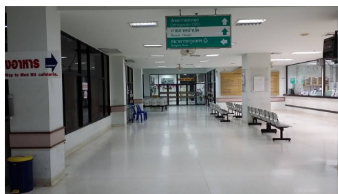
Figure 18. The current condition of the corridor intersection in front of the entrance to the Orthopedic Surgery department
