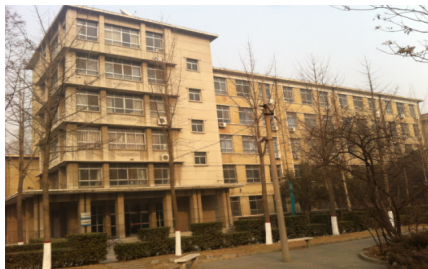
Fig. 1. Five layer brick-concrete structure
