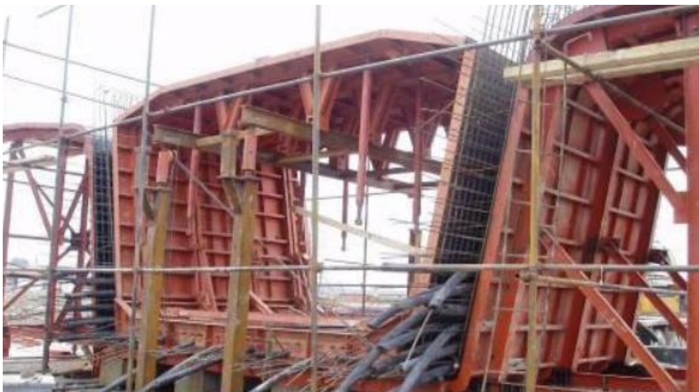
Fig. 6. Formwork installation construction drawing
